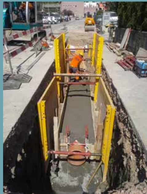
Work being done along Via alle Zocche
